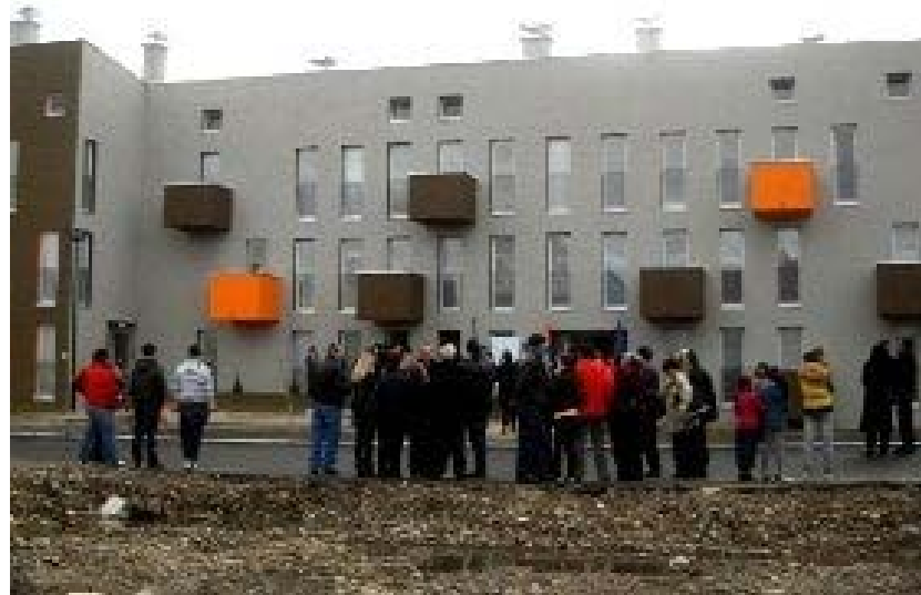
The buildings with 20 apartments
