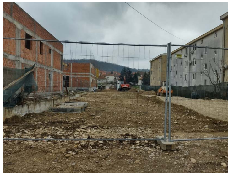
Construction of a nursery in the neighborhood
